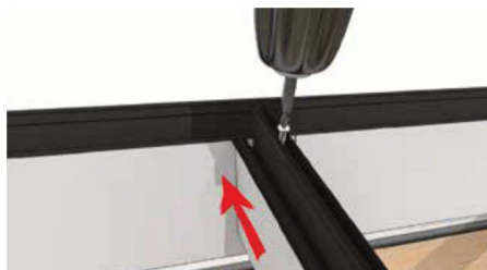
14 Re-tighten the screw in the top of the transom rafter which will pull the joint together and secure.
