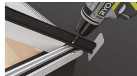
10 Fix hips into the ringbeam using the 4.2 x 25mm screws on either side of the rafter as shown.
